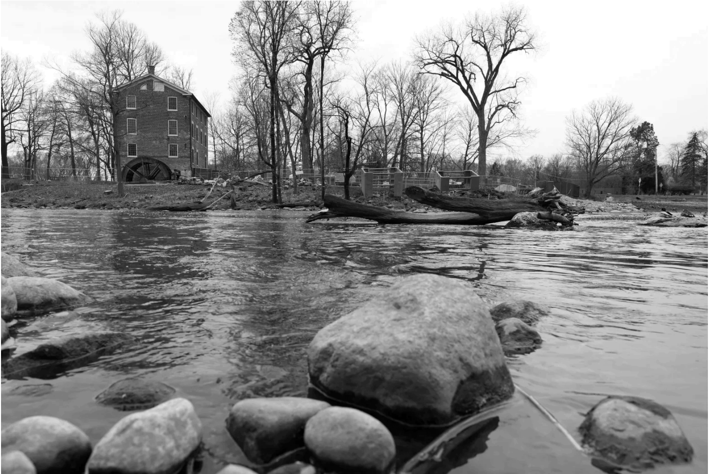
Construction equipment near the area of the former Graue Mill dam on April 11, 2024, in Oak Brook, as part of the Fullersburg Woods and Salt Creek Restoration projects. (John J. Kim/Chicago Tribune)
